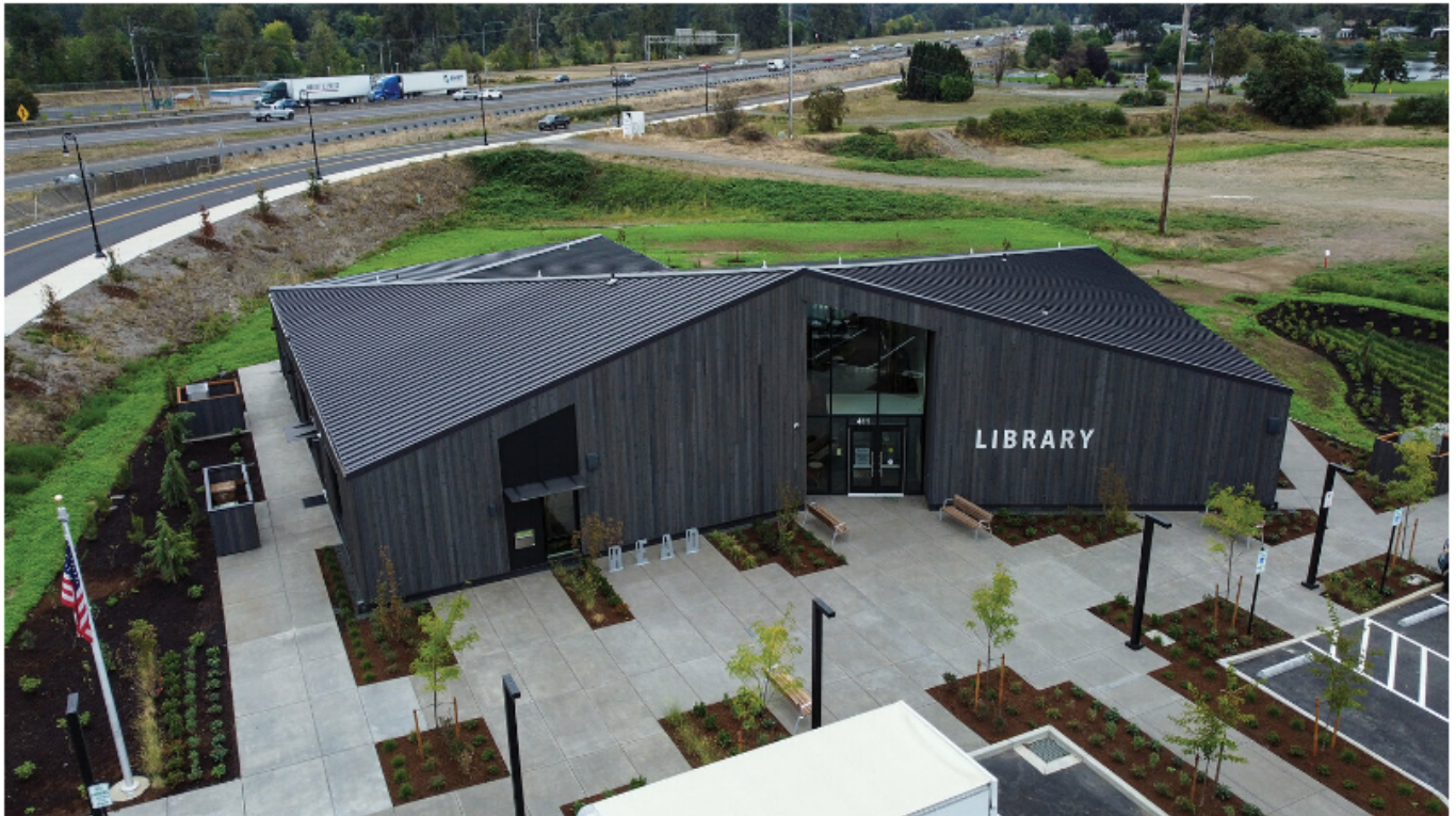
The new Woodland Community Library is a 7,560-square-foot facility located at 411 Lakeshore Drive. The community celebrated its grand opening on Saturday, Oct. 12.
